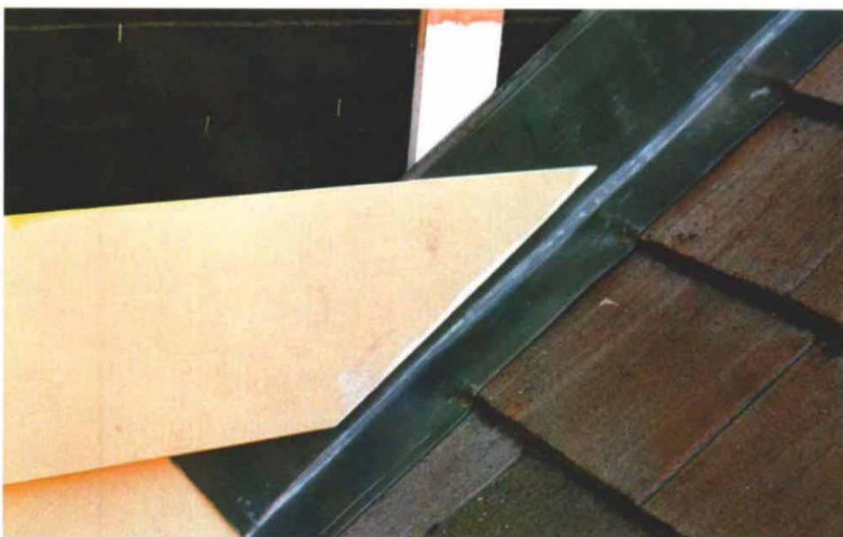
**Counterflashing covers step flashing, Ice & Water Shield and tar paper.** The counterflashing is layered over the lower clapboard to drain, while the upper clapboard stops above it to defeat capillary action.
