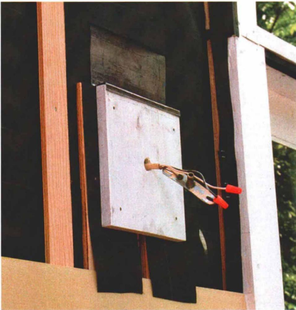
**If siding leaks at joints, let it drain.** The tar-paper splines under this light-mounting block both cover the furring strips and extend over the next lower clapboard to drain water away from the house.
